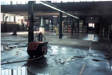
Final Cleaning plus coating.
