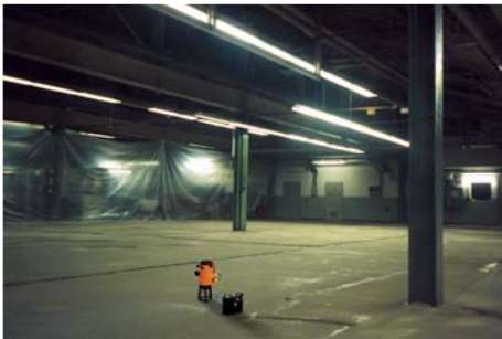
Surface ready for final VAP 1® ORS-C coating.
